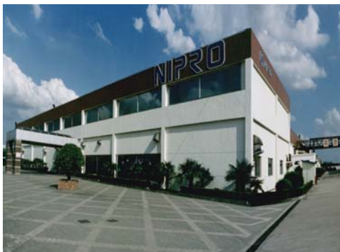
Nipro (Shanghai) Co.,Ltd. Shanghai Plant
